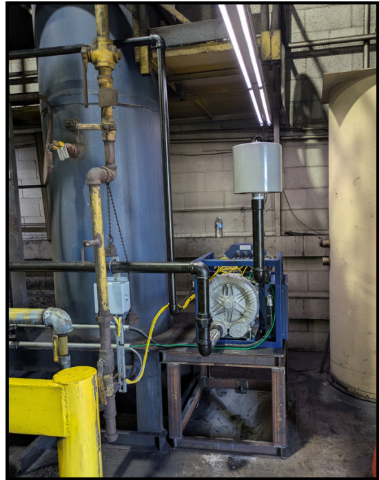
VFD controlled air blower and built-in flow control
