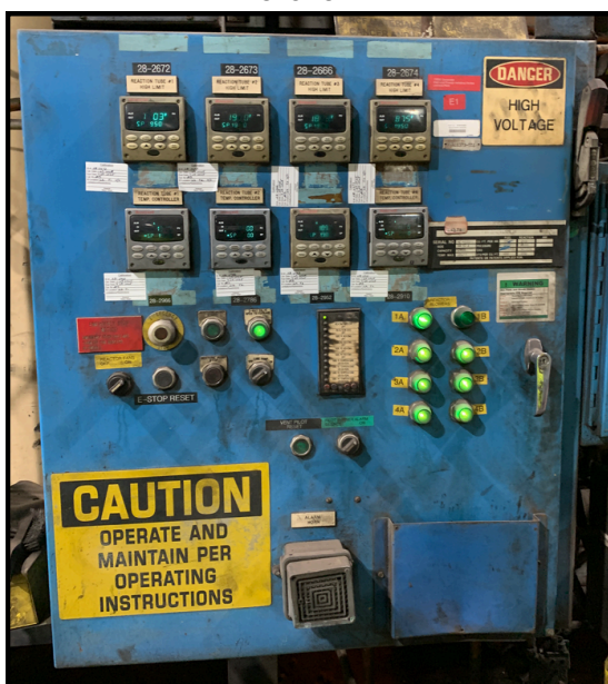
Discrete temperature controller for each tube
